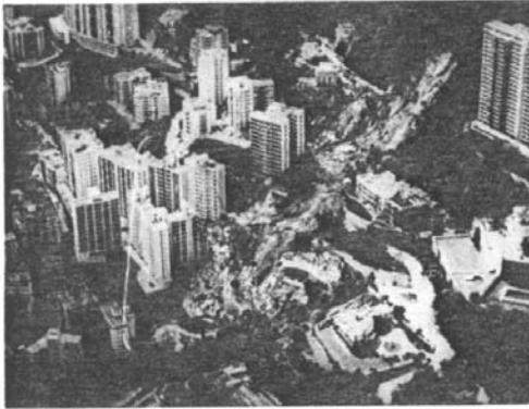
CATASTROPHIC SLIDES, RISKS , DAMAGES, PROBABILITIES e.g. HONG-KONG .
