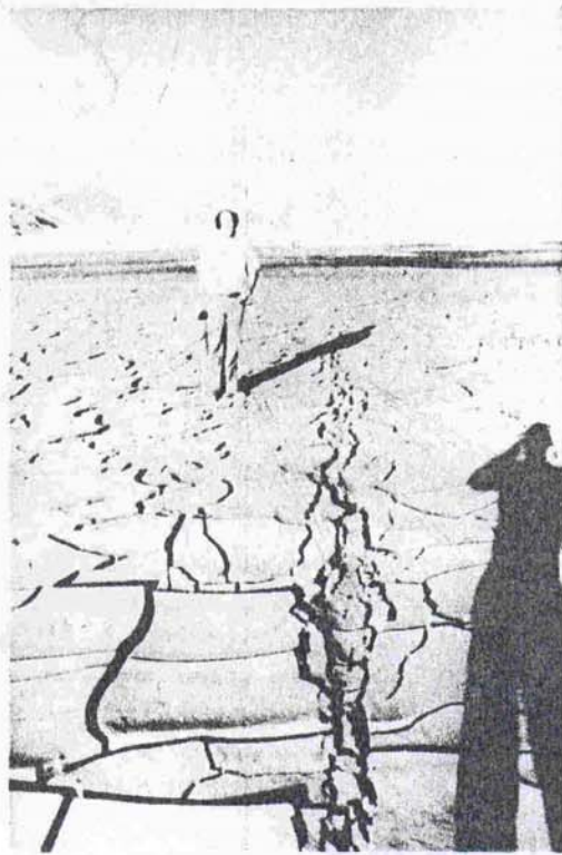
5 a - TYPICAL SINKHOLE INDICATING APPARENT PUNCHED SHEAR .FEW HUNDREDS OBSERVED IN BLANKET WHEN RESERVOIR EMPTIED BY FAILURE
