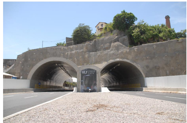
Figure 16. The tunnel concluded
