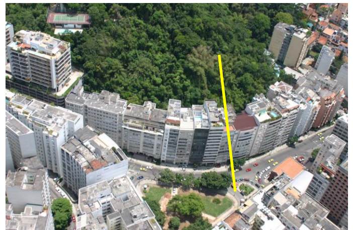
Aerial View of buildings above access tunnel
