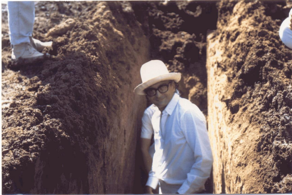
7 - Victor inspecting the compacted fill in Massingir, Mozambique
